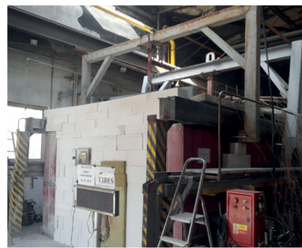
REINFORCED CONCRETE PROTECTION
